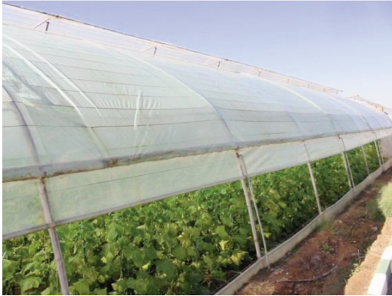
Fig. 4 - Aeration valves are usually not covered with netting by greenhouse owners and this allows the entry of insect vectors.
