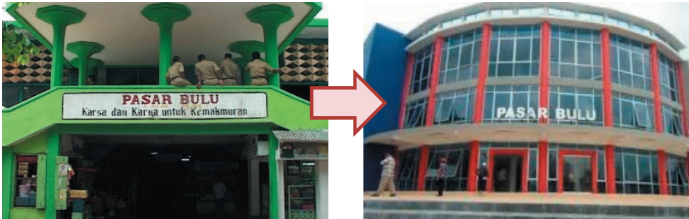
Figure 3. Bulu Market pre-revitalization (left) and post-revitalization (right).
