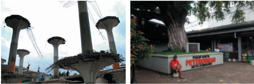
Figure 6. Original column of Bulu Market (left) and Tamarind tree of Peterongan Market (right).
