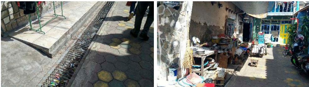
Figure 12. The condition of Bustaman village drainage channel.
