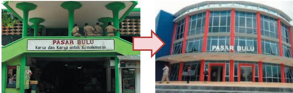
Figure 3. Bulu Market pre-revitalization (left) and post-revitalization (right).
