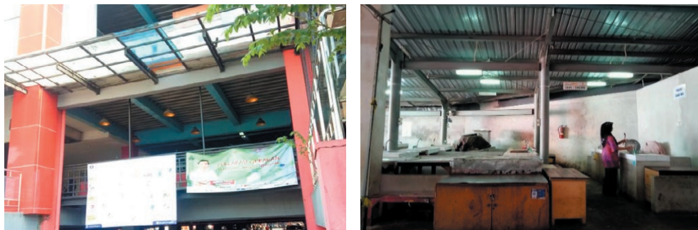
Figure 5. Roofing material for Bulu (left) and Peterongan Markets (right).
