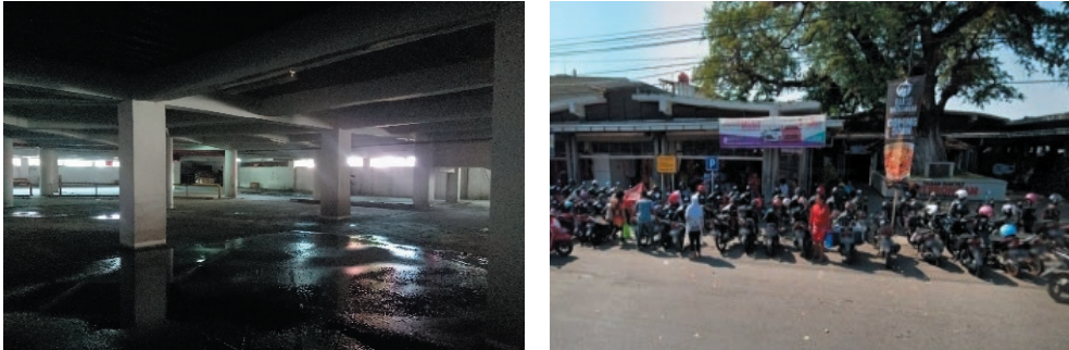
Figure 11. Basement parking space at Bulu market (left) and roadside parking at Peterongan market (right).
