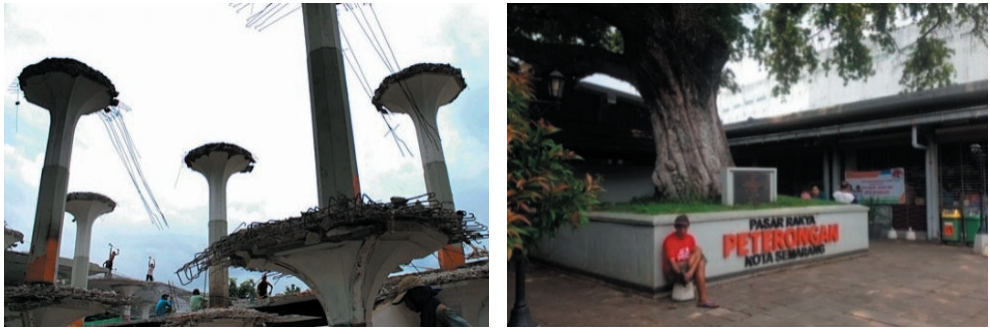
Figure 6. Original column of Bulu Market (left) and Tamarind tree of Peterongan Market (right).
