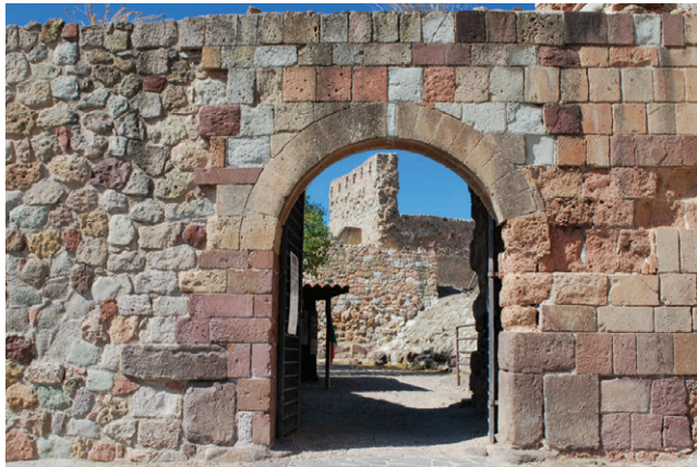
01 | Bosa, Serravalle castle, particular of the fortified wall in volcanic rock ashlars
