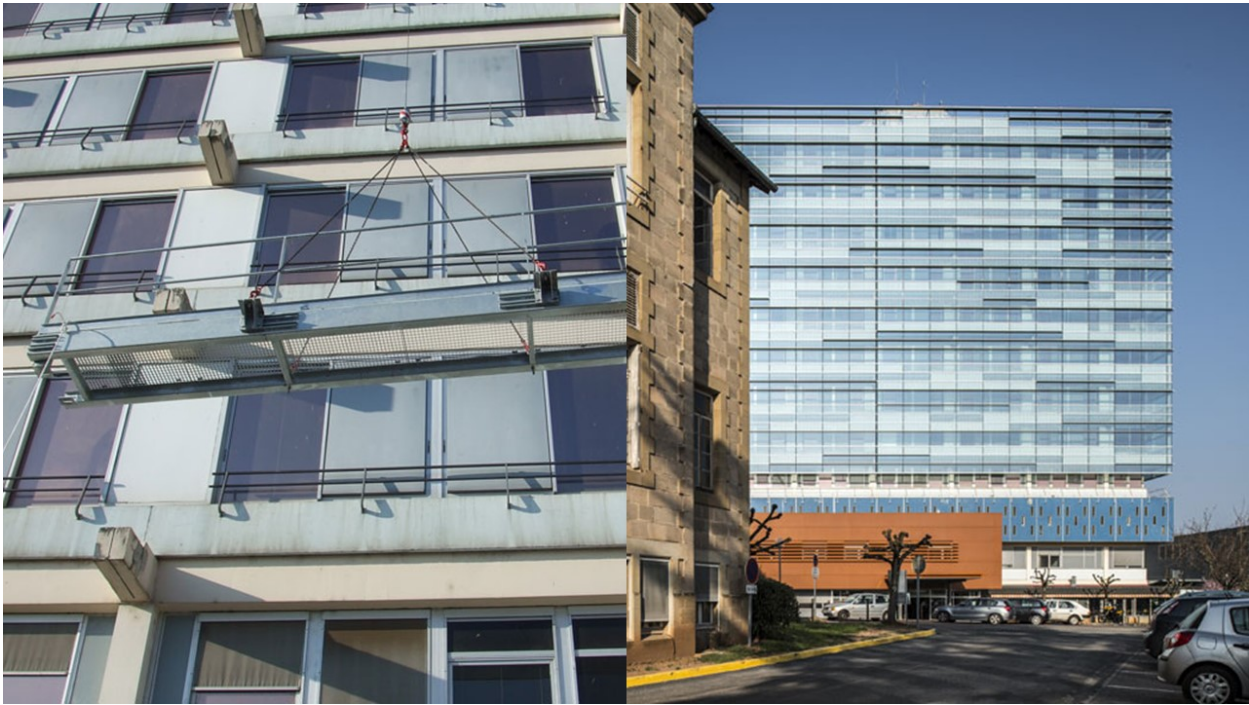
Fig. 1 Brive-la-Gaillarde Hospital, built in 1977 (left picture), and renovated by Vincent Espagno (Espagno Milani Architects) in 2014 (right picture), using a ventilated double-skin facade. Credits: Espagno Milani / Sylvain Mille
