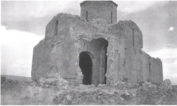
Fig. 6 The deteriorated condition of Mren Cathedral, 1990s (Photo: WMF)
