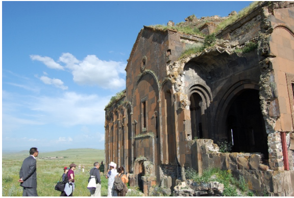
Fig. 2 WMF's Technical Control Team inspecting damage of Ani Cathedral, 2009 (Photo: WMF)
