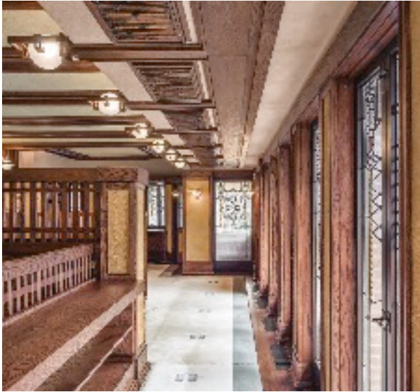
Fig. 4 Robie House, Chicago, the indoor level of reconstruction in the wooden finishes, the light devices, the window frames, 2019, Harboe Architects.
