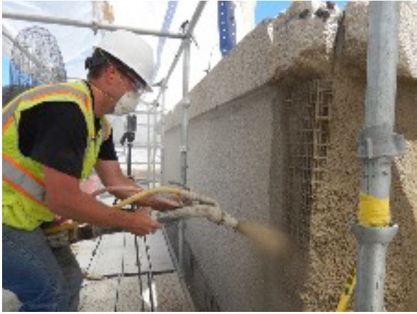
Fig. 2 Unity Temple, Chicago, the grid metal reinforcement placed in the outdoor elevation in the recent restoration works, 2015, Harboe Architects.
