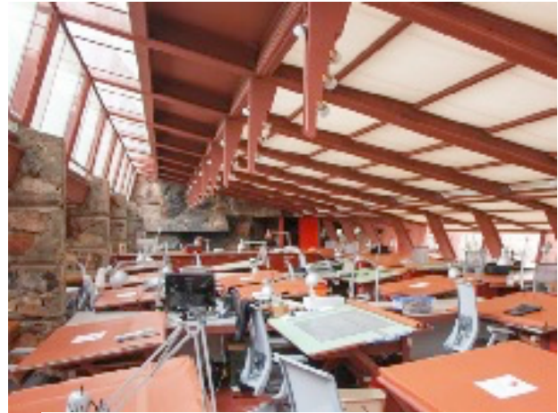
Fig. 7 Taliesin West, Scottsdale, the current studio with the new metal beams, the glass windows and a new lighting system, 2014, inexibit.com.
