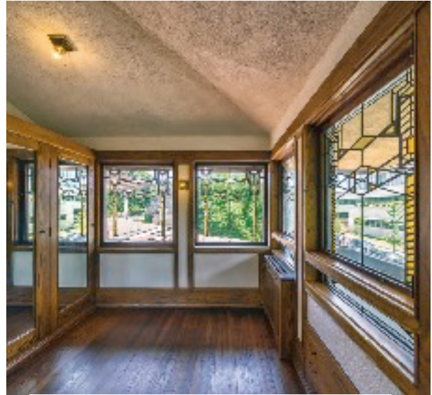
Fig. 5 Robie House, Chicago, the indoor level of reconstruction in the wooden finishes, the wooden floors, the light devices, the window frames, the ceiling rough plaster, 2019, Harboe Architects.
