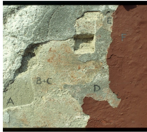
Fig. 4 Casa Malaparte, Coating stratigraphy (source: G.Pertot)
