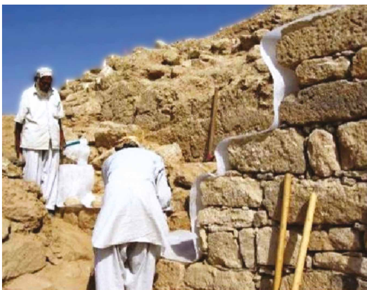
Fig. 13 Examples of some of the procedures proposed for the restoration of the North-East tower of al-Wu'ayra (Sassu, et al., 2012)
