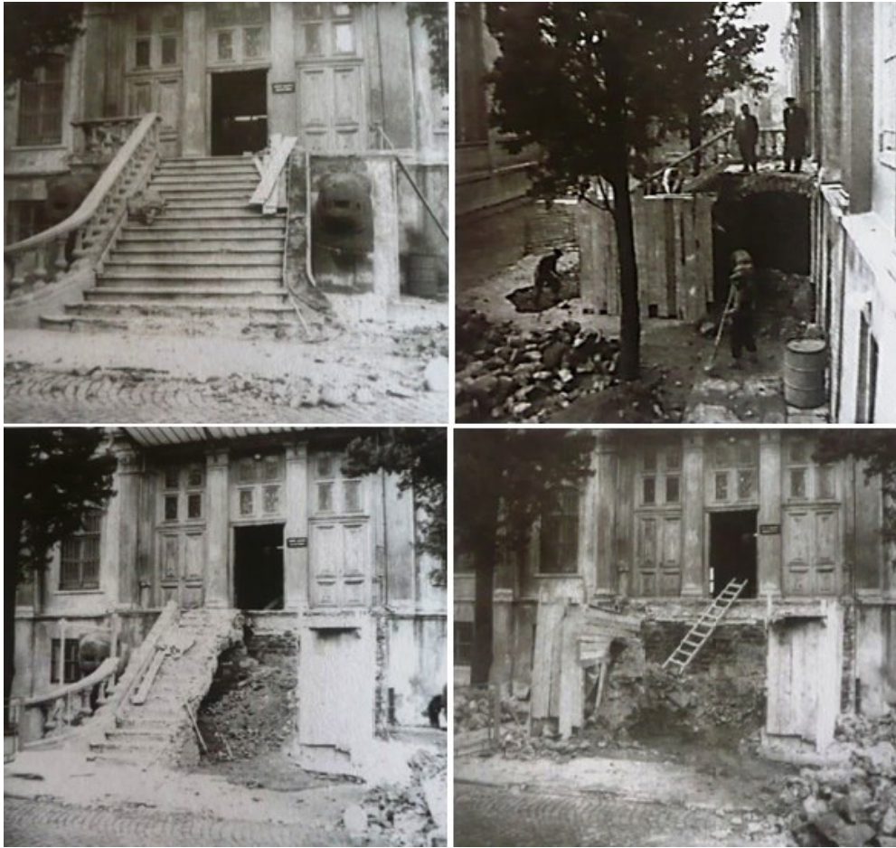
Fig. 6 Demolition of the original staircase and entrance during the 1963-1974 conversion of the Sanayi-i Nefise Mektebi into the Museum of the Ancient Orient (Source: Istanbul Archaeological Museums Archive, Istanbul Directorate of Surveying and Monuments Archive, Council for the Conservation of Cultural and Natural Property Archive, 1998).
