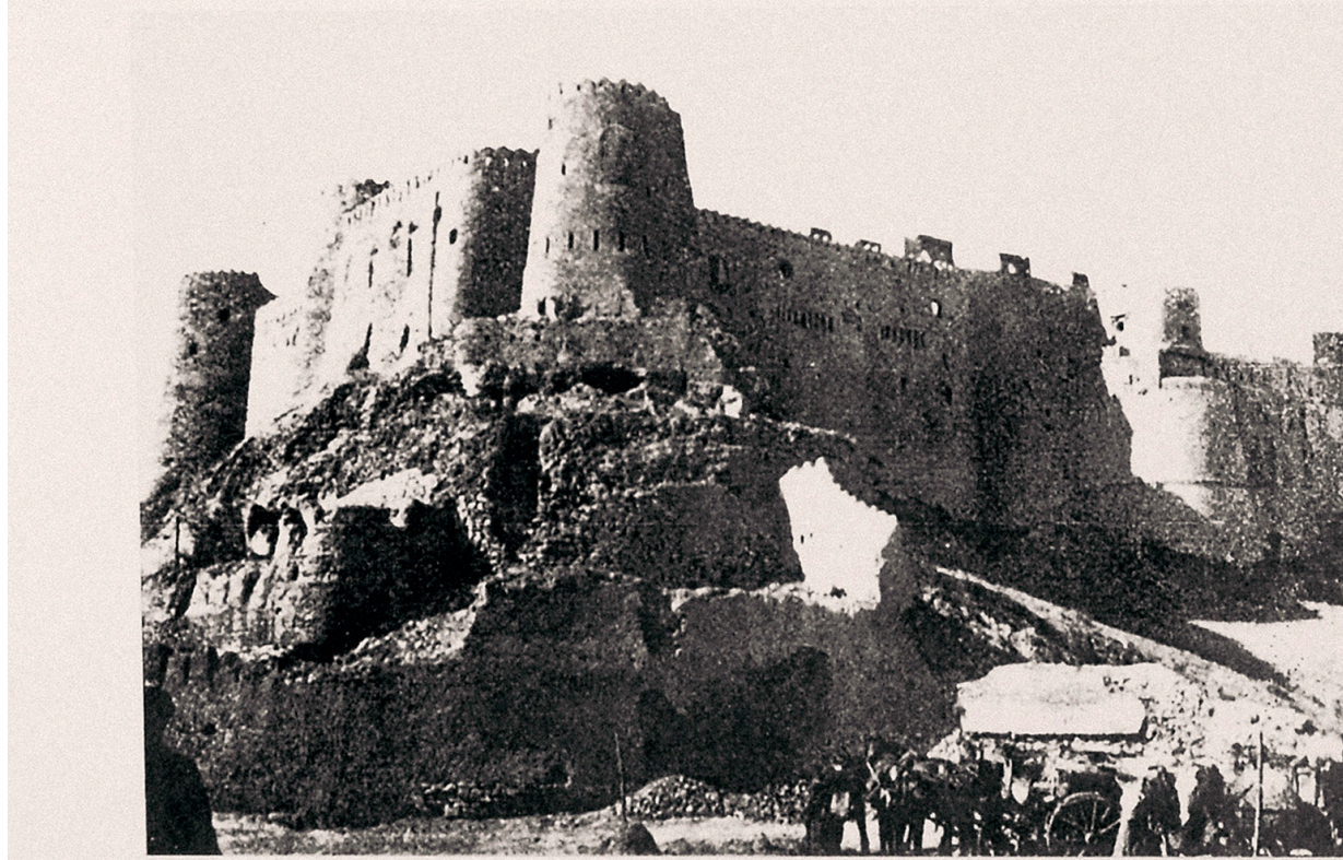
20.3 Herat, the fortress' north-eastern wall (1975)
