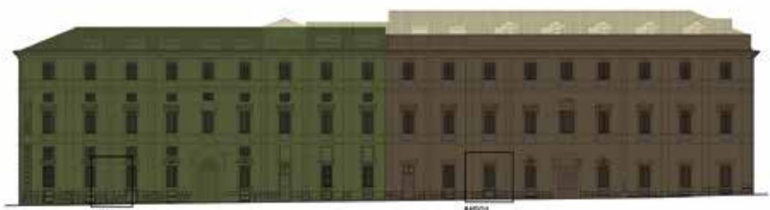
The East façade
