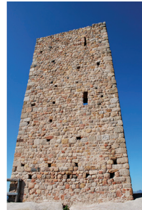
02 | Olbia, Pedres castle, particular of the tower in granitic rock ashlars
