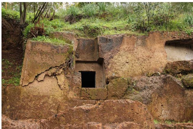
Figg. 19-22 Several situations in which the lignified roots of tree and shrub species have produced severe damage to artefacts
