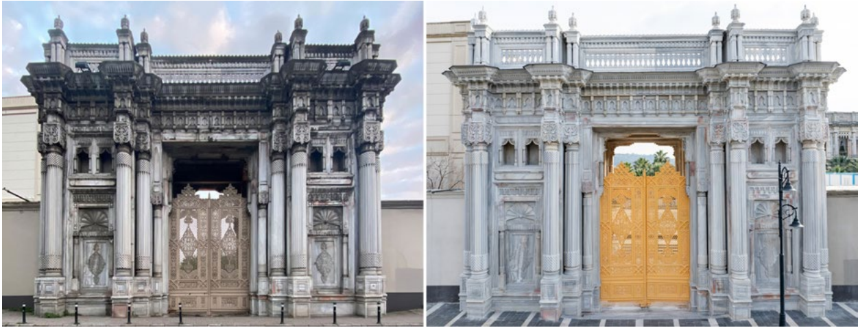
Figure 1. Sultanate Gate, Road Facade, before and after (photo F. Betül Değirmenci Breitenfeldt, 2022-2023).
