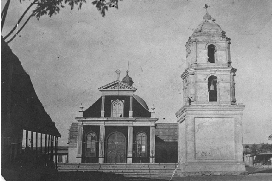
Figure 4. Matilla Bell Tower. Photograph taken at the beginning of the twentieth century, used as reference for the restoration of the dome in the 1950s. (Photograph obtained by Roberto Montandón Paillard. Archivo Fotográfico del Consejo de Monumentos Nacionales).
