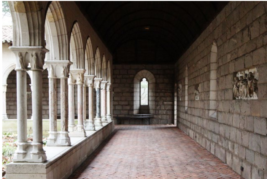
Figure 1. New York, the MET Cloisters, One of the outdoor courtyards with spolia fragments arbitrarily recomposed in the construction of the complex in 1935 (Photo by Davide Galleri, 2024).
