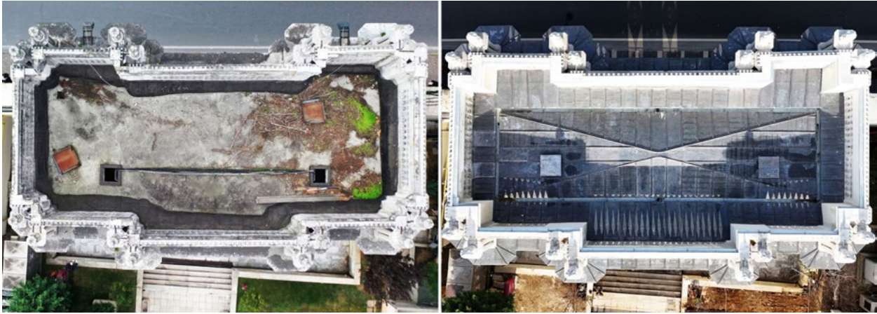
Figure 2. Application of new lead-covered timber roof (photo F. Betül Değirmenci Breitenfeldt, 2023).
