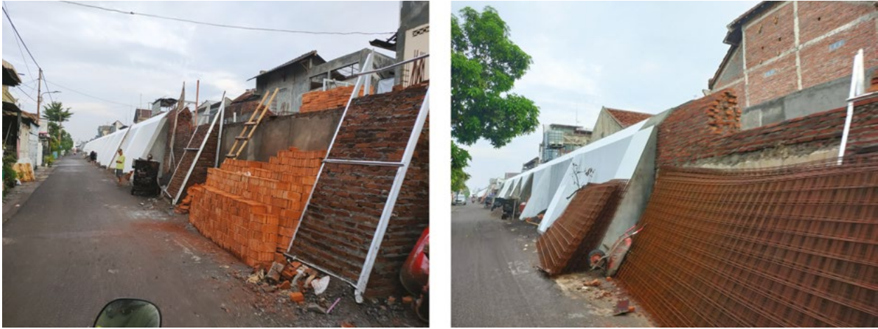
Figure 4. Reconstruction of Baluwerti wall system on Yogyakarta's palace complex that uses modern materials and methods which undermines the authenticity of the historical property (photographed with collaboration with A. Lestaringtyas, 2023).
