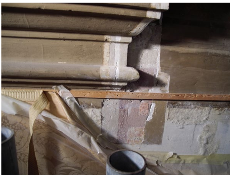
Figura 4. Rome, Embassy of the United States of America, entrance room to the Ludovisi building, stratigraphic test through exposure window: sequence of decorative layers after the 17th century (photo Giartosio, 2021).
