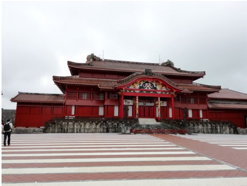
Figura 4. Naha, Shuri-jō Castle, the state hall before the fire in 2019 (Photo J. Mukai).
