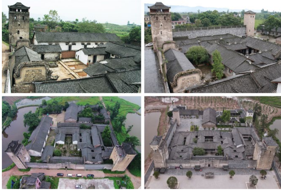
Figure 4. The Shi-Pai-Fang House: before restoration (left, 2014 © Archive of Luxian Cultural Heritage Administration, Sichuan), and after restoration (right, photo P. Jiang, 2023).
