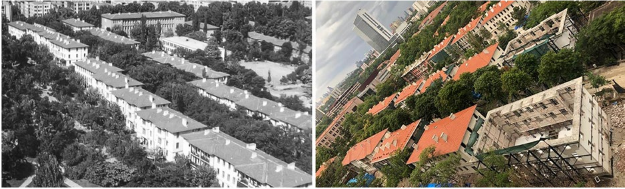
Figure 1. Ankara, Saraçoğlu Neighborhood, Paul Bonatz, 1944 (© VEKAM Archive, Ankara, open access TKV0981_01; left), designated in 1979, transformative reuse project, 2019-2023 (photo C. Kılıççöte 2022; right).
