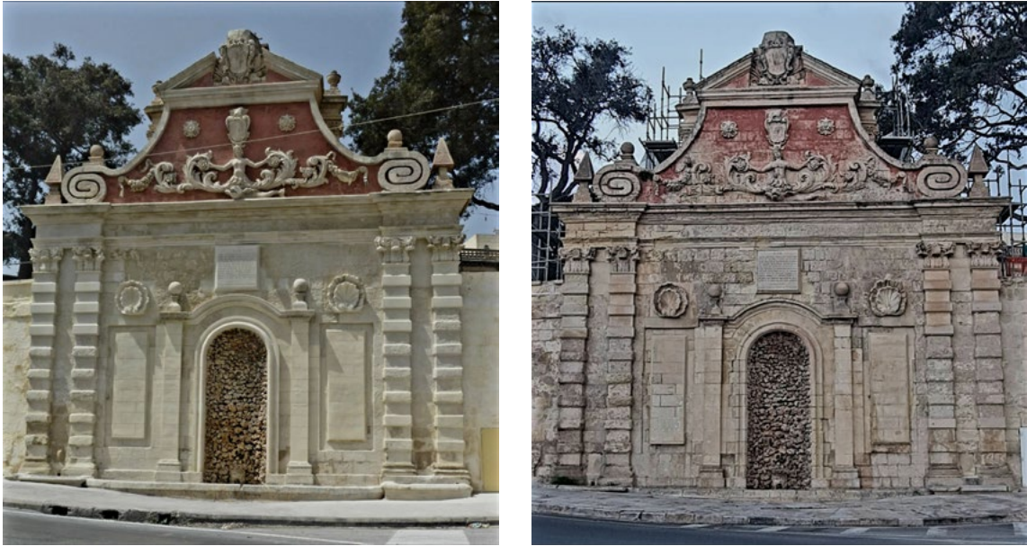
Figure 1. Saqqajja Fountain, Mdina, after restoration (left) in 2010 and 14 years later (right) in 2024 (image RPD, 2024).
