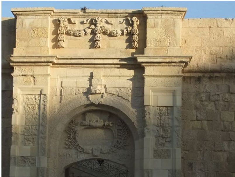
Figure 3. St John's Bastion, Vittoriosa, after restoration in 2012 (image RPD, 2012).
