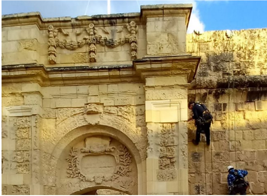
Figure 4. St John's Bastion, Vittoriosa, ongoing maintenance in 2024 (image RPD, 2024).
