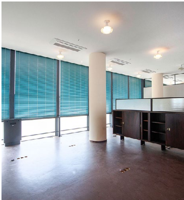
Fig. 3 Rio de Janeiro, Gustavo Capanema Palace. The south façade and its blue blinds. Details of the air conditioning already installed between the pillars and the linoleum flooring (photo by O. Liberal, 2025).
