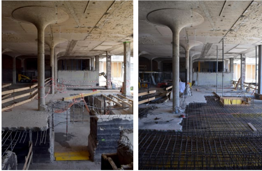
Fig. 7 Zurich, Intensive demolitions and structural interventions within the Kongresshaus Los I area, while still respecting the original mushroom column and flat slab structures designed by Robert Maillart, (photo by P. Fleming, 2018).
