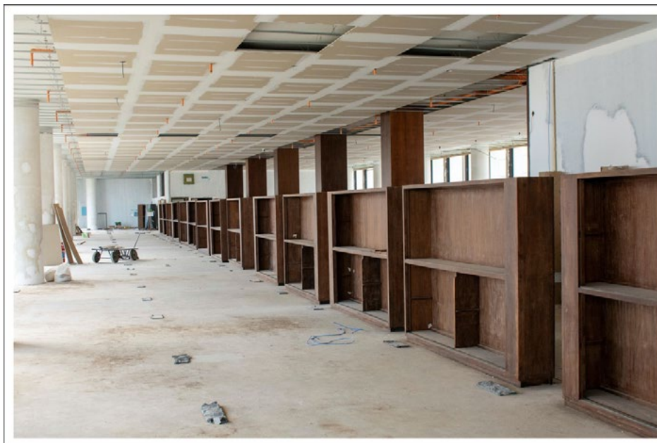
Fig. 2 Rio de Janeiro, Gustavo Capanema Palace. Details of the cabinets where the air conditioning was supposed to be installed previously, and of the 15 cm false ceiling being made for its installation (photo by O. Liberal, 2023).
