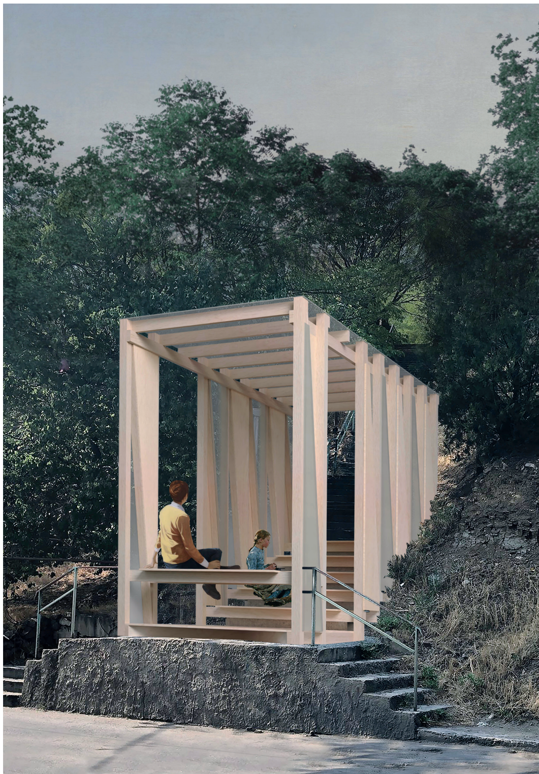
Fig. 9 –Pavilion Common Steps, a punctual intervention for regenerating urban landscape. View from the street. 2020 (Author copyrights: NOIA practice)
