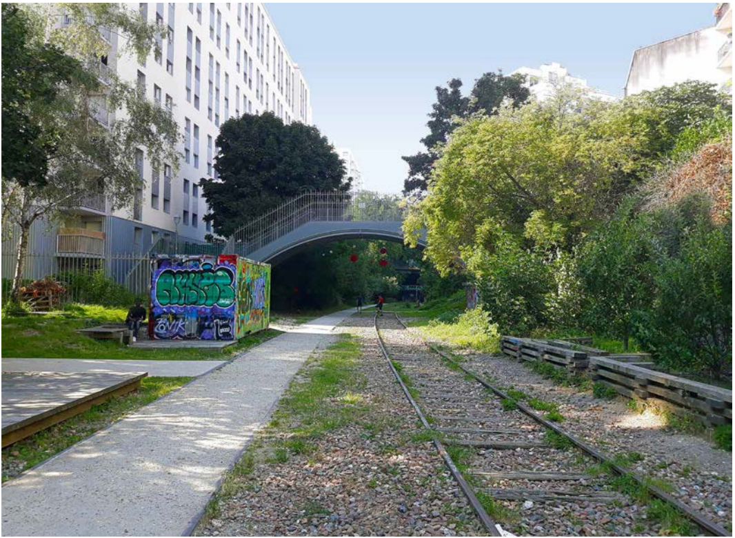
Fig. 5 - The container and the small space for passive recreation (photo: Manuela Ronci, 2021).
