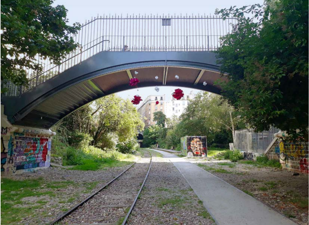
Fig. 3 - Passerelle de la Mare, Paris. The footbridge crosses the railway cutting (photo: Manuela Ronci, 2021).
