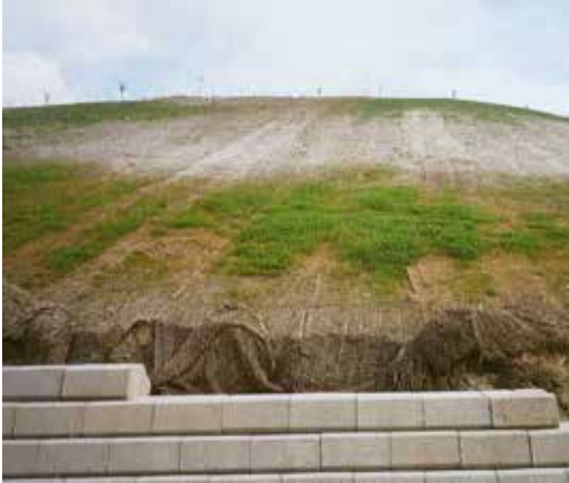
Fig. 10 – Slope with an anti-erosion mesh of jute fiber in the Valdemingómez Forest Park, after the recovery (source: Madrid Council).
