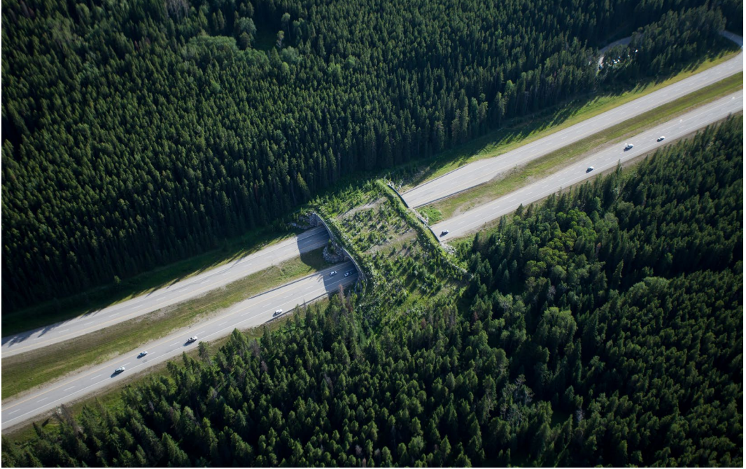
Image Credit: Yellowstone to Yukon Conservation Initiative. Animal crossing overpass, Banff National Park, Alberta. Photo © Paul Zizka Project Credit: The Yellowstone to Yukon Conservation Initiative is a joint Canada-United States not-for-profit organization dedicated to securing the long-term ecological health of the region. See https://y2y.net/ .
