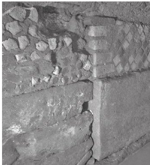
Fig. 6 – Detail of the Cloaca Maxima masonry at the intersection with the Sacra via collector. On the upper left, the Republican or Augustan age restoration of the Roman Kingdom conduit (bottom part); on the right, the connection of the Imperial age conduit (E. Bianchi).
