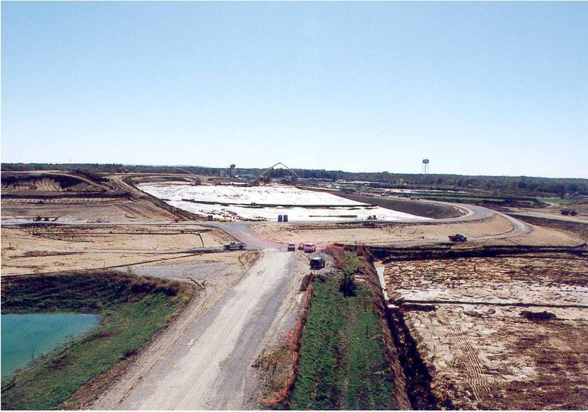
**Fig. 2** – Grout manufactured at the Chemical Stabilization and Solidification Plant is piped directly on and around the waste in the Disposal Cell (photo: Energy Government, 10 May 2002).
