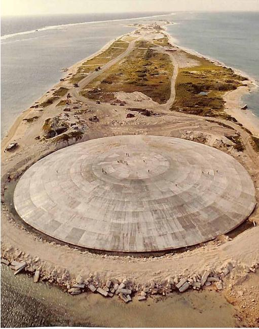
**Fig. 8** – Aerial view of Runit Dome (or Cactus Dome), Runit Island, Enewetak Atoll. In 1977-1980 the crater created by the Cactus shot of Operation Hardtack was used as a burial pit to inter 84,000 cubic meters of radioactive soil scraped from the various contaminated Enewetak Atoll islands. The Runit Dome was built to cover the material (photo: US Defence Special Weapons Agency, 1980).
