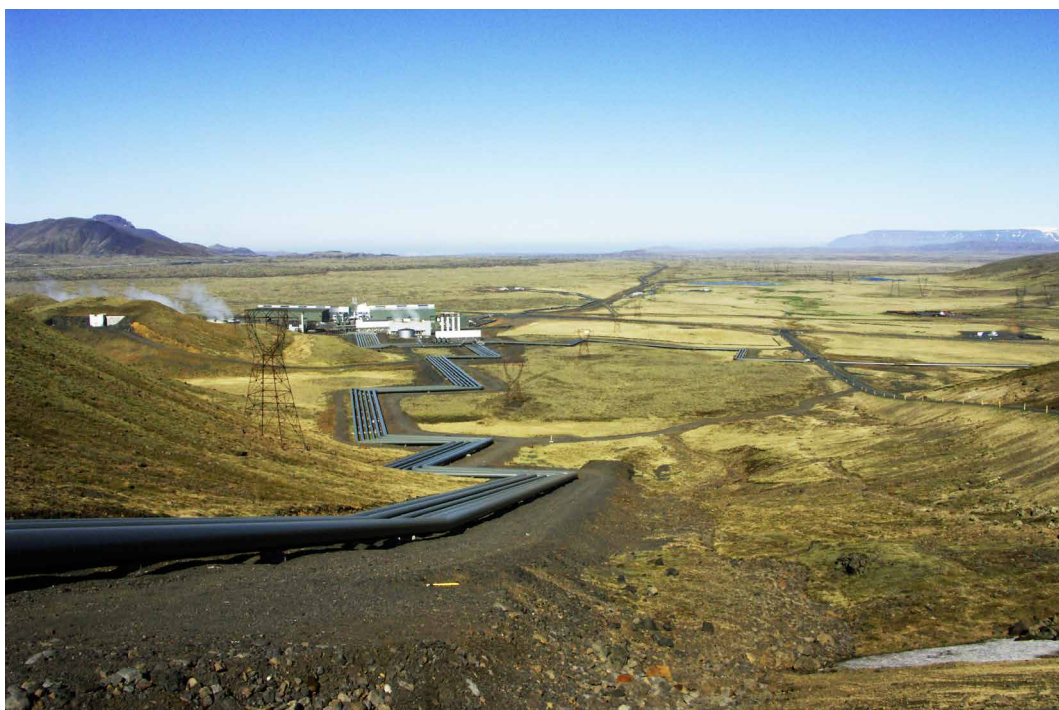
Fig. 14a,14b – The Geothermal pipelines and land reclamation at ON Energy company (before reclamation on top, and after below). (Photo: courtesy Magnea Magnúsdóttir).
