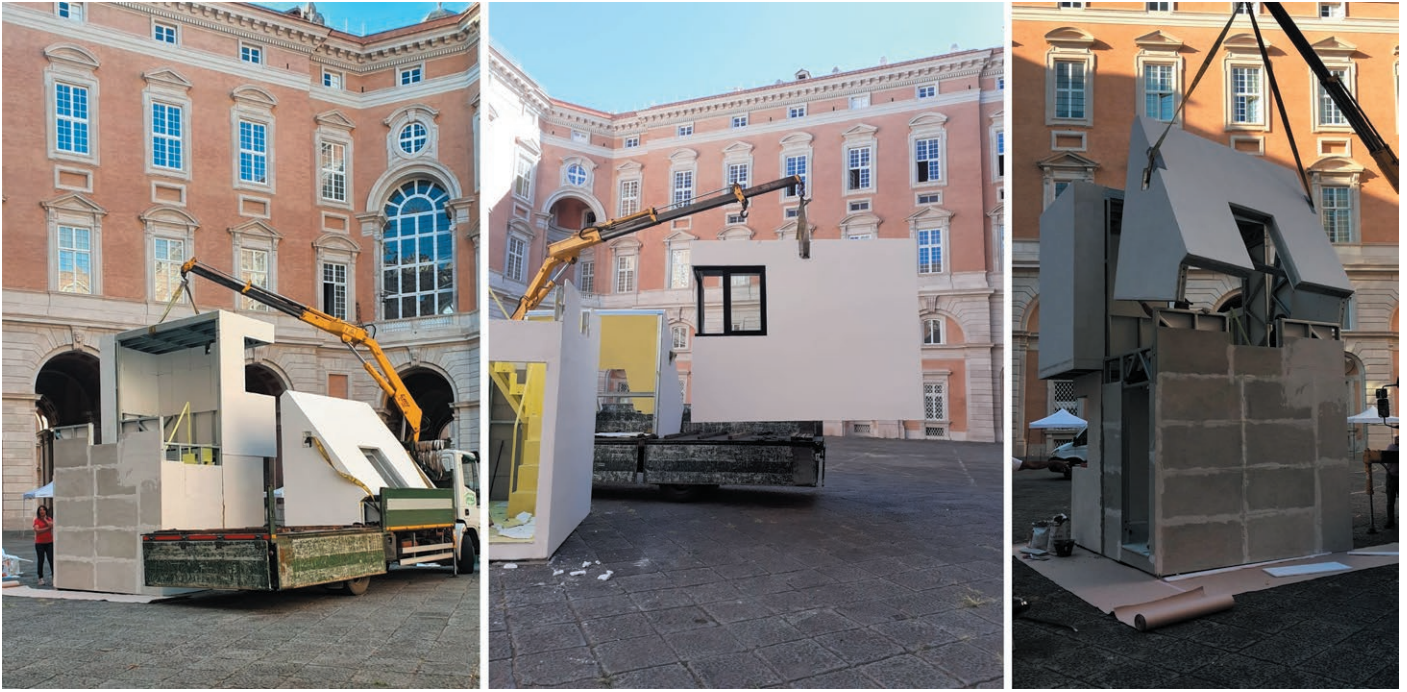
04 | The transport and assembly phase of the prototype
