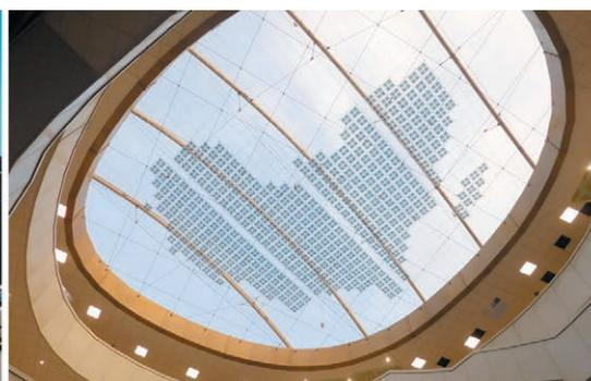
were adopted and, in particular, SunPower Maxeon® cells measuring 125x125 mm.
