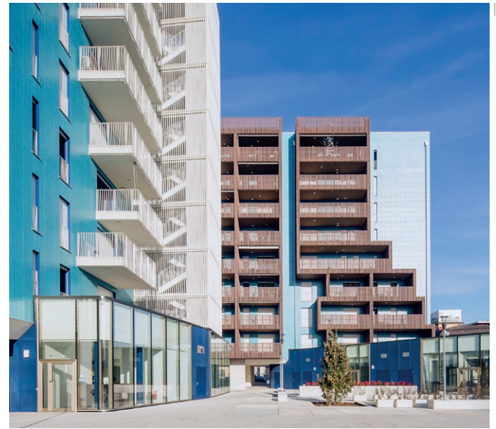
04 | Complesso residenziale "Urbagreen" a Romainville (Francia). Foto ©Stefano Anzini Residential complex "Urbagreen" in Romainville (France). Photo ©Stefano Anzini
