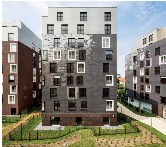
02 | Complesso residenziale "Living in the Blue", Lambrate (Milano). Foto ©Stefano Anzini Residential complex "Living in the Blue", Lambrate (Milano). Photo ©Stefano Anzini
