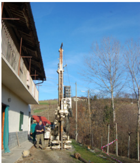
05 | L'edificio durante le indagini geologiche The building during the geotechnical investigations
