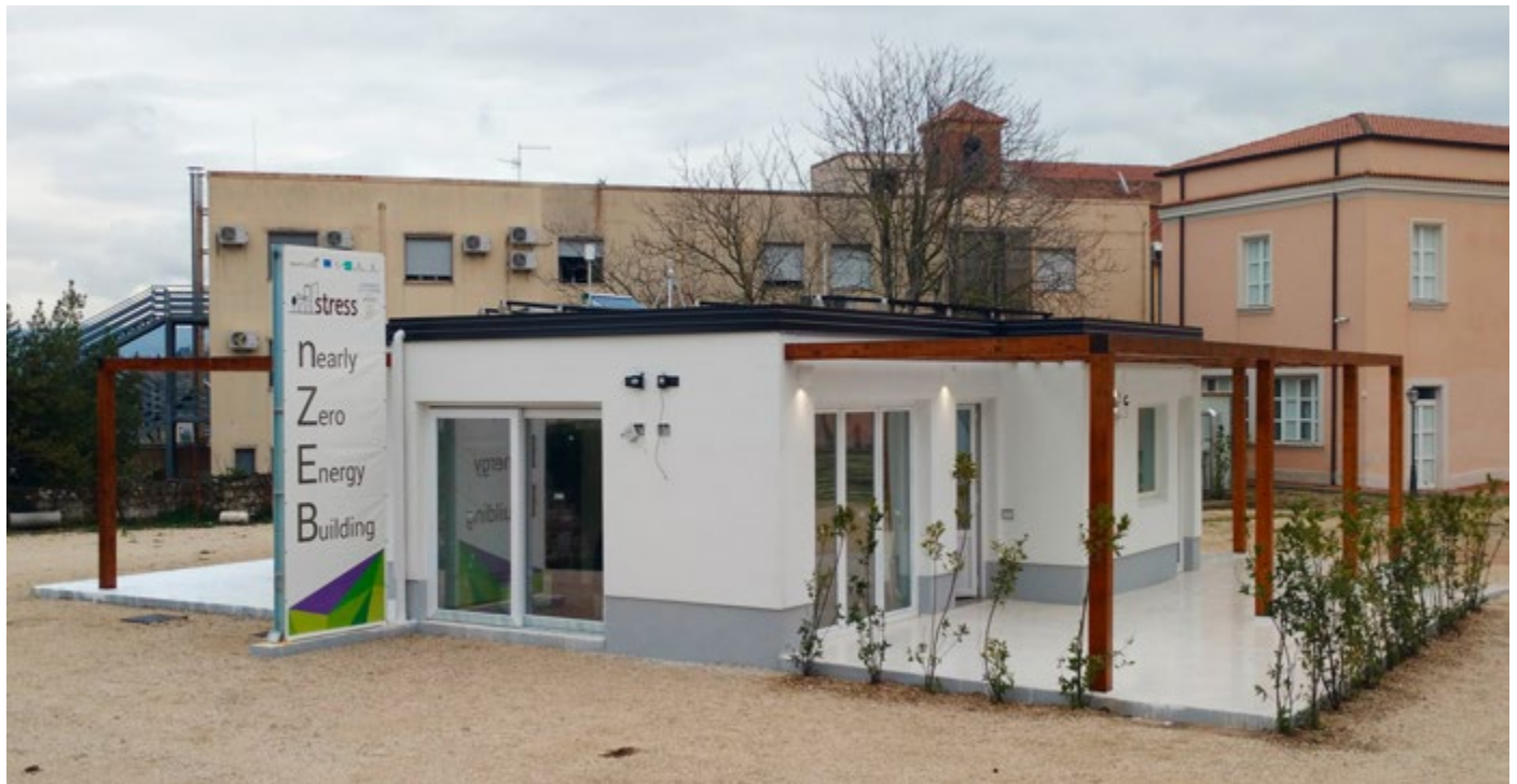
07 | Demonstrator building, Benevento. nZEB near completion
