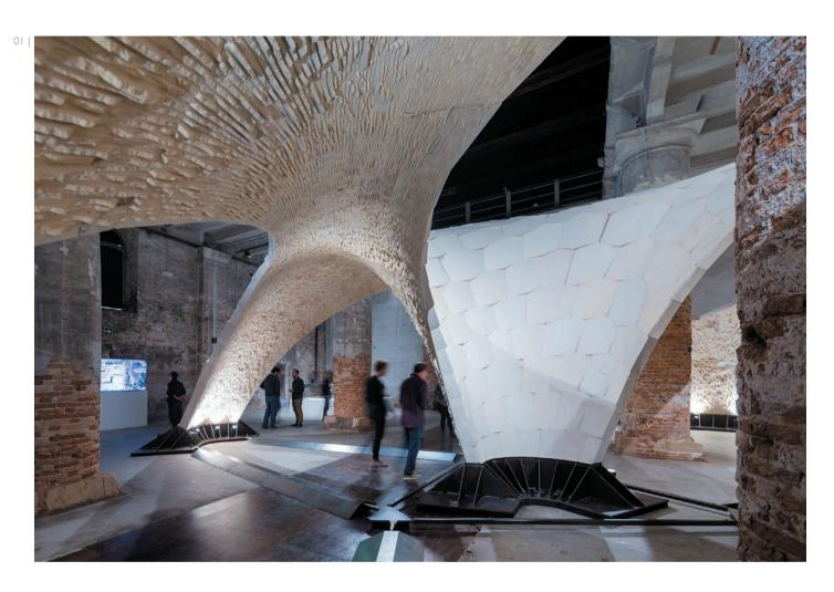
by fabrication constraints to the point that already in the design process, the geometry is defined considering the CNC machining process for the stone cutting, and the on-site assembly (Rippman *et al.*, 2016). Moreover, this vault has been conceived to be assembled and then disassembled after the Biennale and to be re-assembled elsewhere
