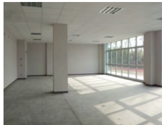
18 | Liceo Scientifico Majorana: Aula completata Majorana School: classroom
