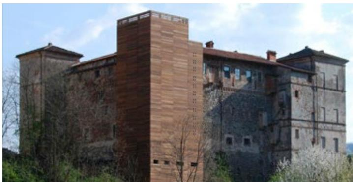
dimensions of the cabin adequate for the expected tourist flow – choosing an external solution, independent also statically from the monument, which has allowed the absence of the subtraction of antique matter (Fig. 4).
