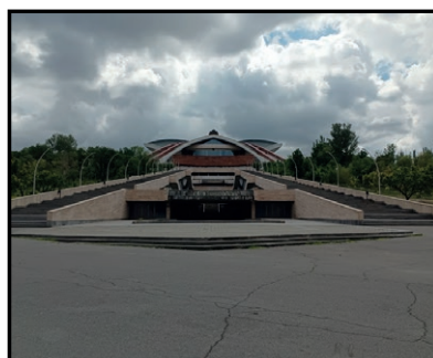
The Demirchian Center staircase between Leningradyan Street and Genocide Memorial Garden
