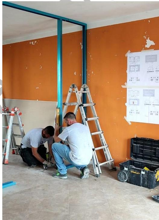
Figure 6. Internal partition monitoring in the construction site-school of Gerenzago
