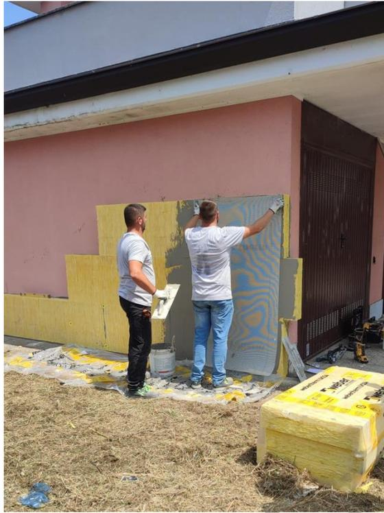
*Figure 7. Installation of a thermal coat in the construction site-school of Gerenzago*
