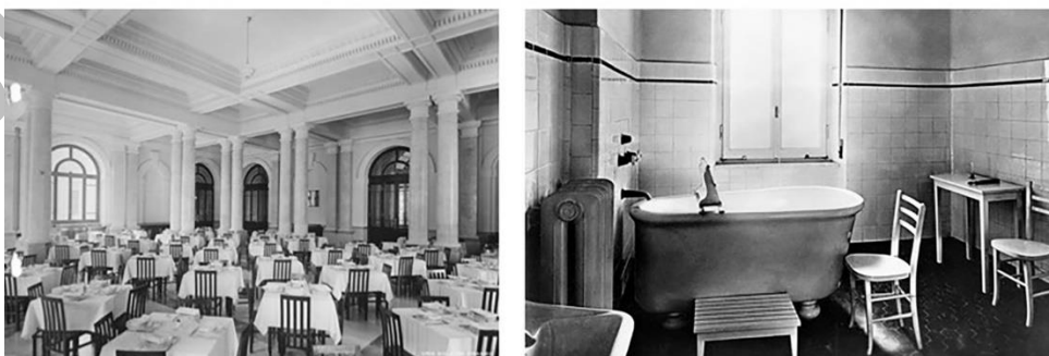
Fig. 03 - Historical images of the complex
