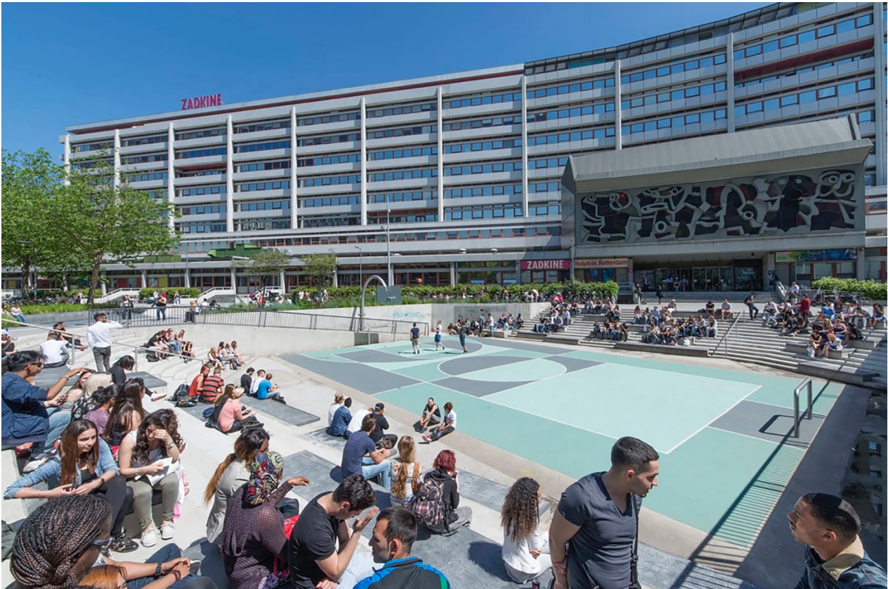
Fig. 04 - Water Square Bentheimplein, Rotterdam. Multifunctional public space used as a recreational and sports area, integrated with a temporary stormwater storage system, Wikimedia Commons.
